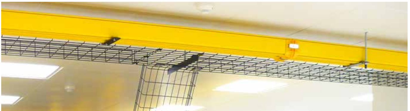
Typical installation of an overhead tray with ceiling mounted supports
