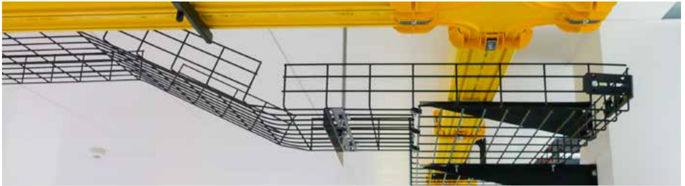
Typical installation of an overhead tray with brackets and support angles
